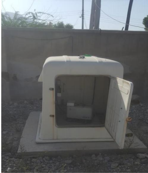
Figure 3. Sياهو station with SSA2 digital accelerometer.
